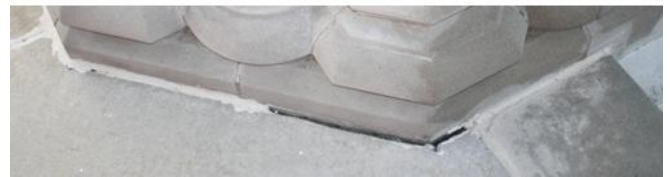
← Bell Tower Vertical Movement Cracks
