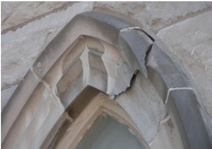
Damage to Stones & Stone Patches
