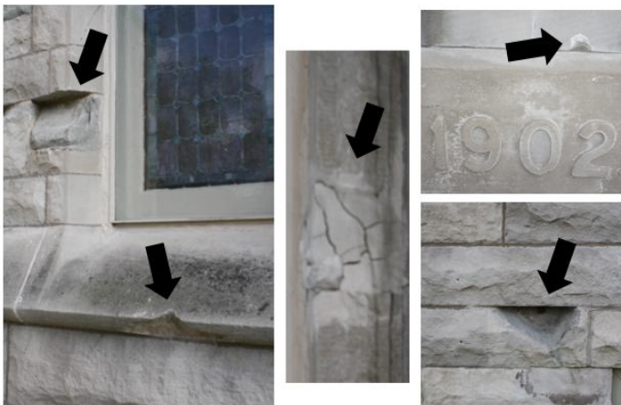
Damage to Stones & Stone Patches
